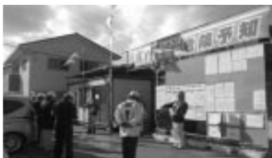
(大串定住促進住宅工事現場)
