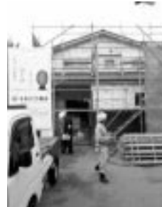
(前野邸工事現場)
