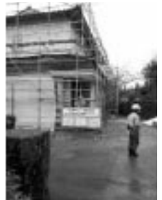
(湯浅邸工事現場)
